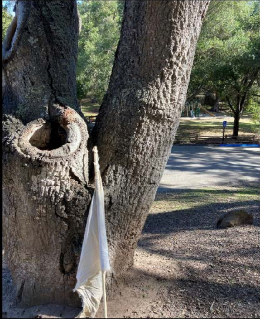
View of the tree hole in the trunk of this oak tree.
